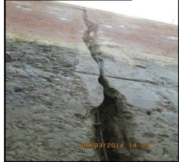
Monolith Joint Deterioration
